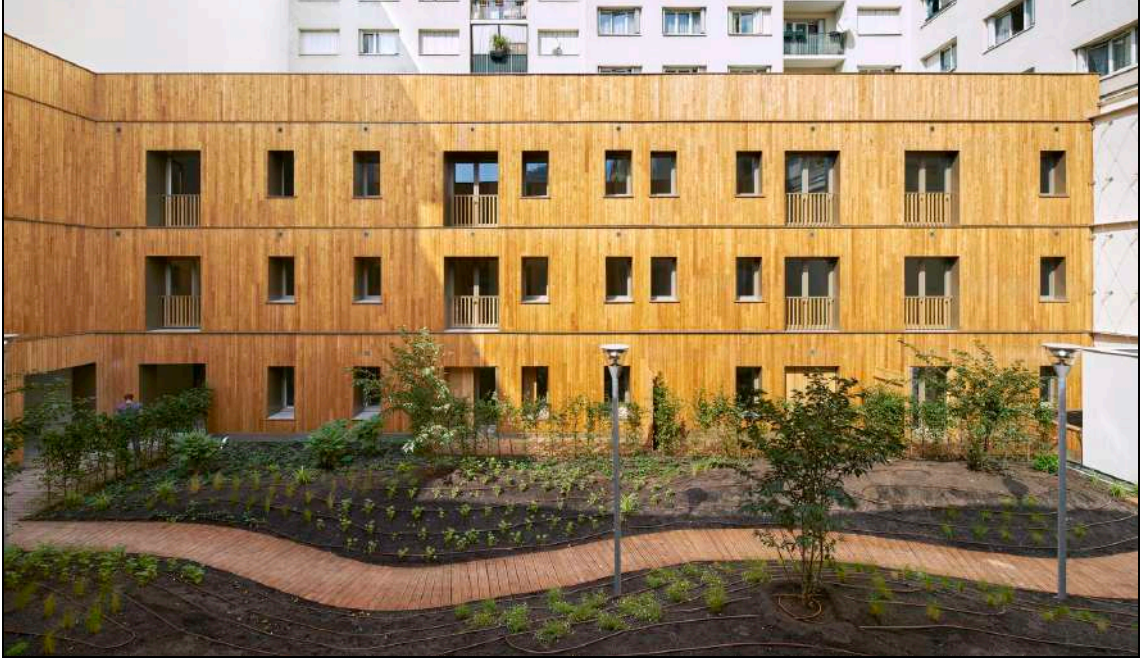
Şekil 3.12. 90 Housing And Office Avluya Bakan Cephe (URL-7)
