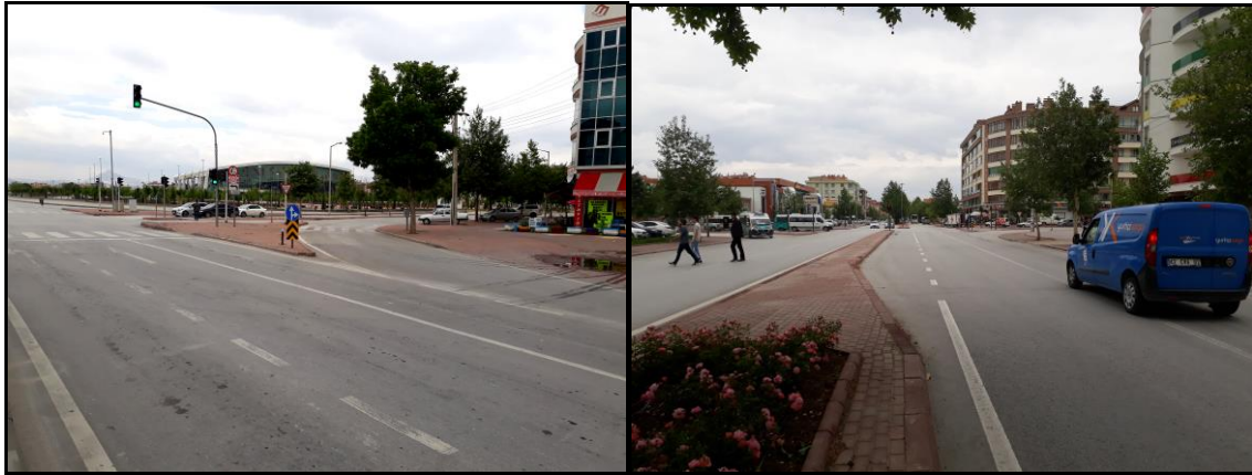
Figure 2.17 Flared and channelized intersection, Konya (Personal archive, 2018)
