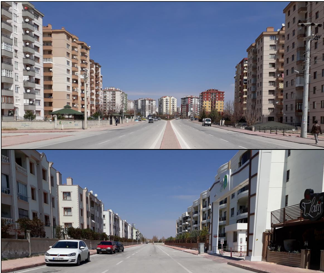
Figure 4.14 Identical building facades, zones 2 and 3 (Personal archive, 2019)
