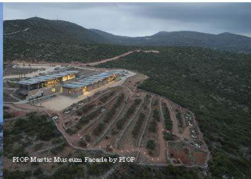
PIOP Mastic Museum Facade by PIOP
