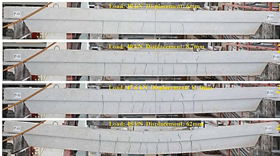
Fig. 7. Damage history of P-0.
