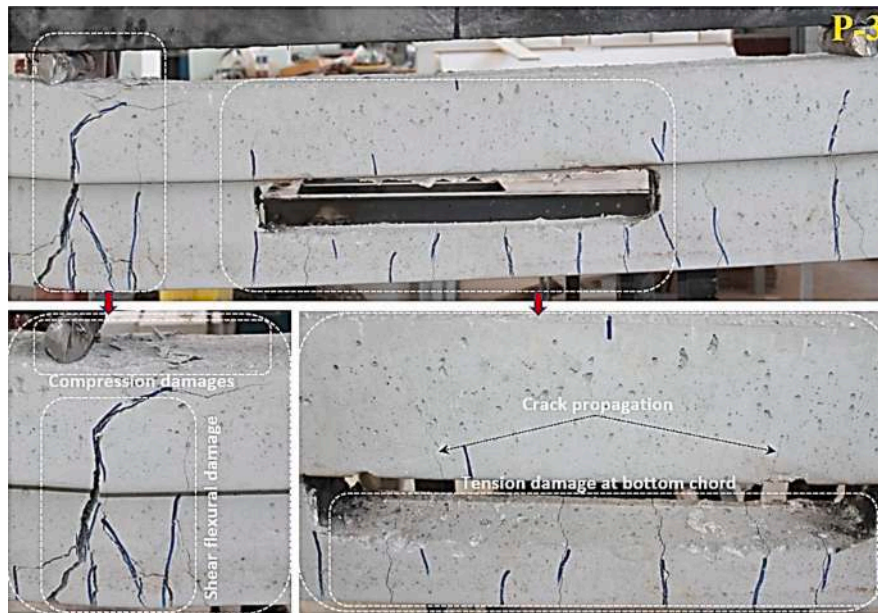
Fig. 10. Damage analysis of P-3.
