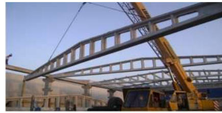
Fig. 1b. Prefabricated reinforced concrete hollow rafters
